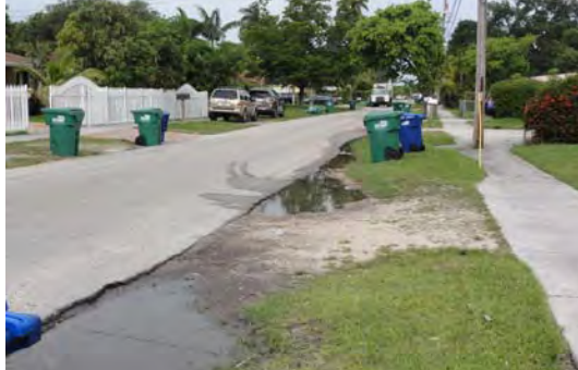
Swales in Arch Creek Estates look tired and no longer offer stormwater management.
