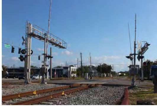
The site for the proposed Tri-Rail Coastal Link station is surrounded by a low density of uses, providing an opportunity for housing and economic development.
